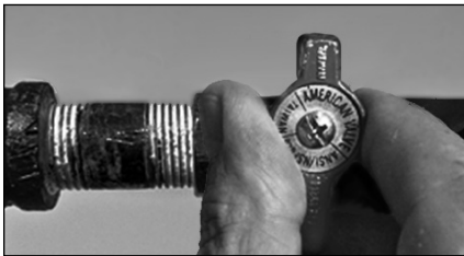
Figure 50 - Gas valve in “off” position.
